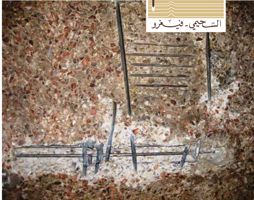
Spalled surface affected by heating exposing pre-stressed tendons.
