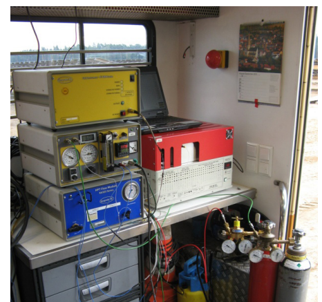
MIP controller and gas detector units.
