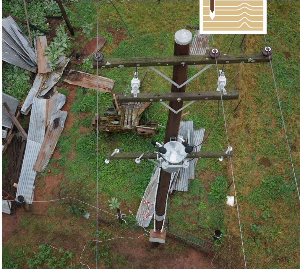
Improved and prioritised workforce mobilisation for maintenance.
