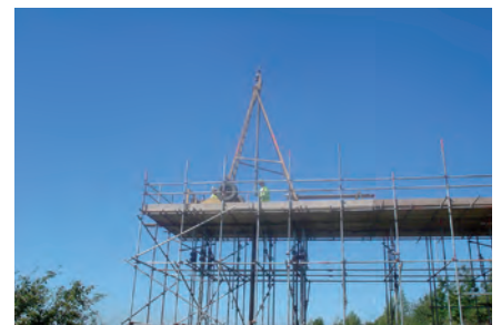
Working off a scaffold platform.
