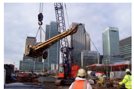
Craned to location.
