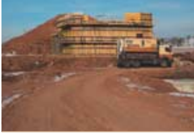
Cone Penetration Test for the foundation of a bridge near Roßla, Germany.
