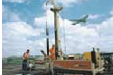
Soil investigation near Schiphol airport.
