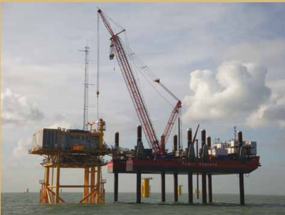
▲ Fugro Seacore's jack-up barge, Excalibur at Thanet
