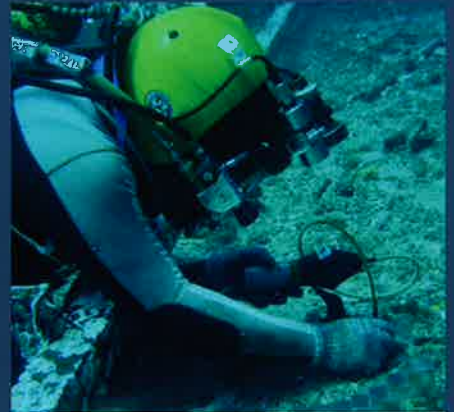
▲ Fugro Brasil Diver performing NDT inspection
